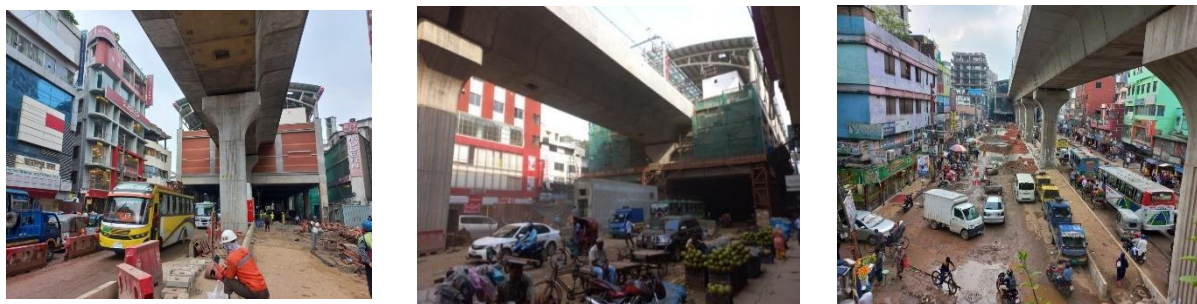
Figure 15: Road Blockage Due to MRT Line 6 Construction
